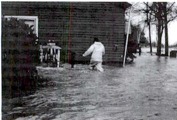
Flood waters from Des Moines Creek surrounded buildings at the Senior Center.
