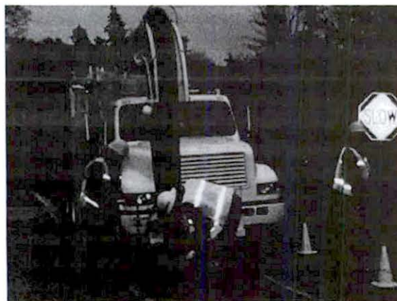
The City vactor truck at work cleaning a storm drain.
